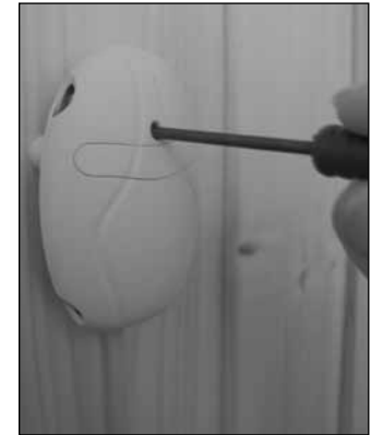
Figure 11. Reset button for overheating limiter
